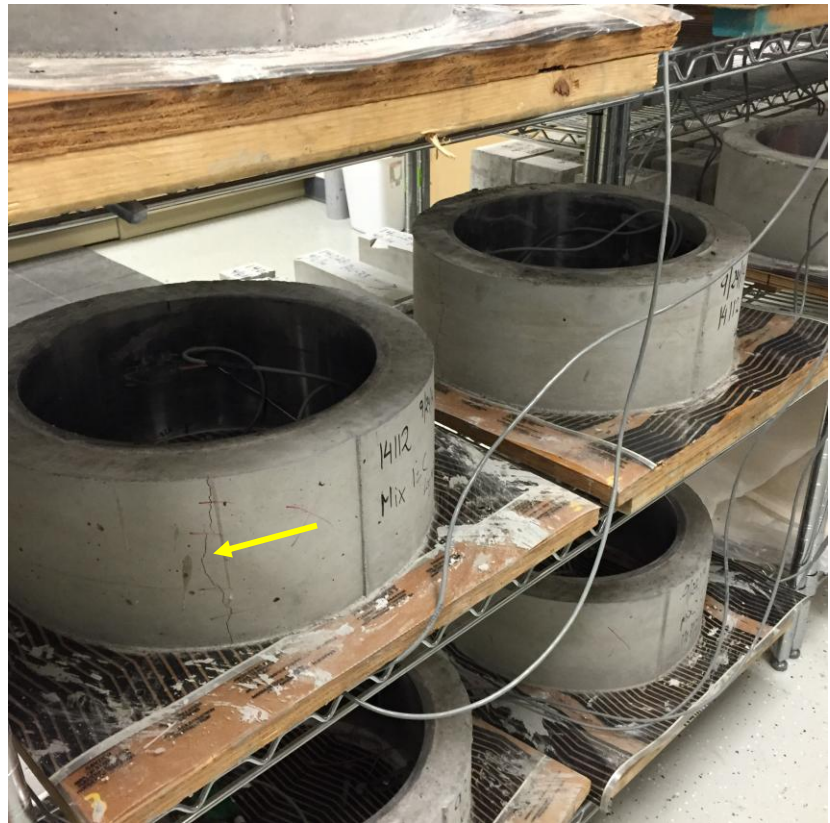
Rings in testing with ring on top left cracked due to drying shrinkage.
