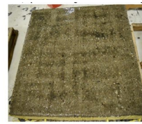
e) First coat of epoxy application
