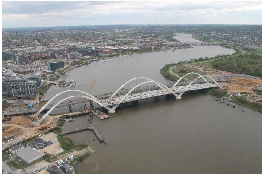
Construction of Frederick Douglass Memorial Bridge
